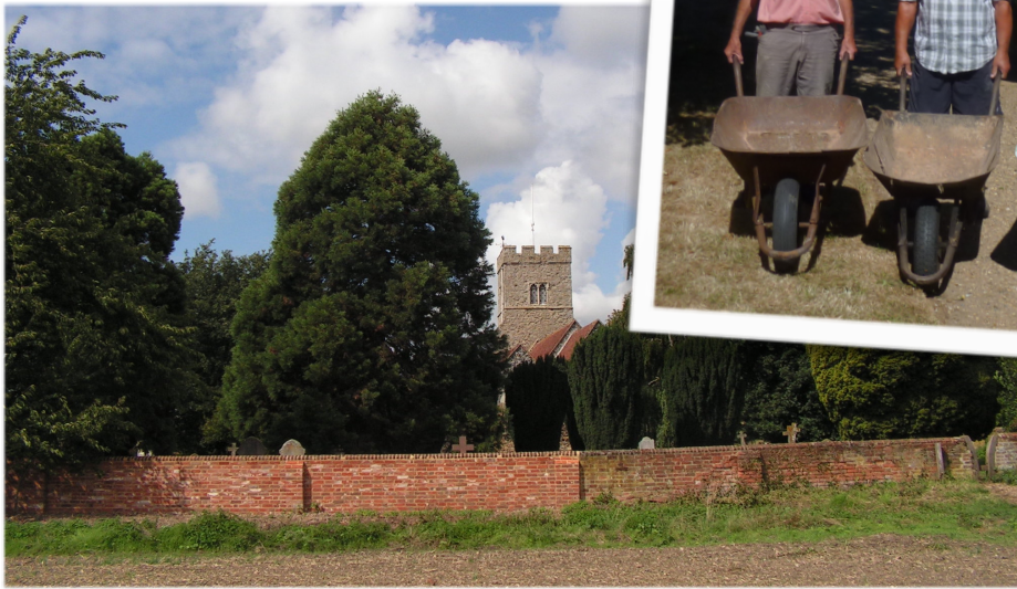
The finished wall in all its splendour
